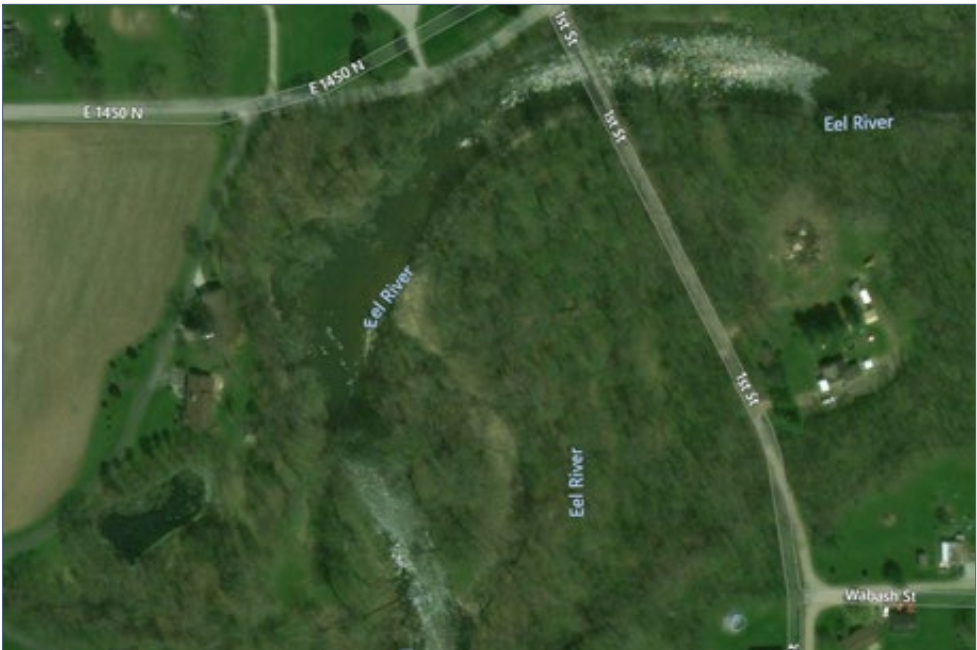
FIGURE 2.8-14 | Liberty Mills Dam after removal, 2016
