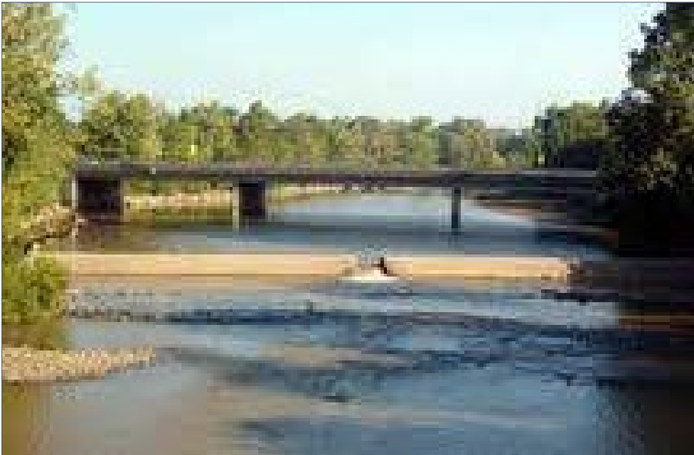
FIGURE 2.8-47 | Central Avenue Dam before removal, 2007
