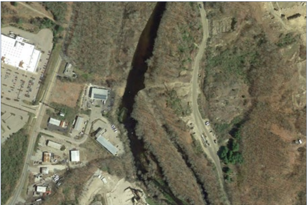
FIGURE 2.8-10 | White Rock Dam after removal, April 2016
