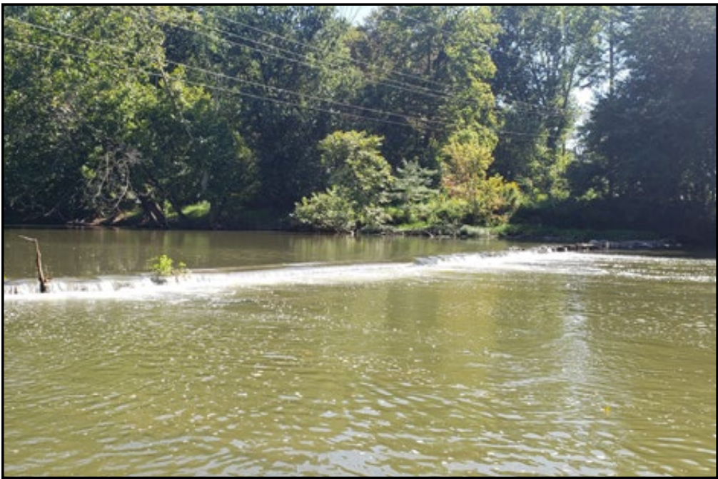
FIGURE 4.6-2 | Piqua Water Company Dam
