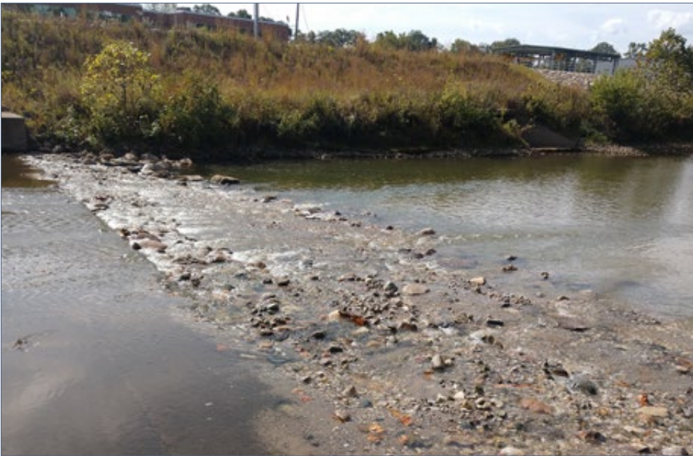
FIGURE 2.8-43 | Completed constructed riffle. October 10, 2019.
