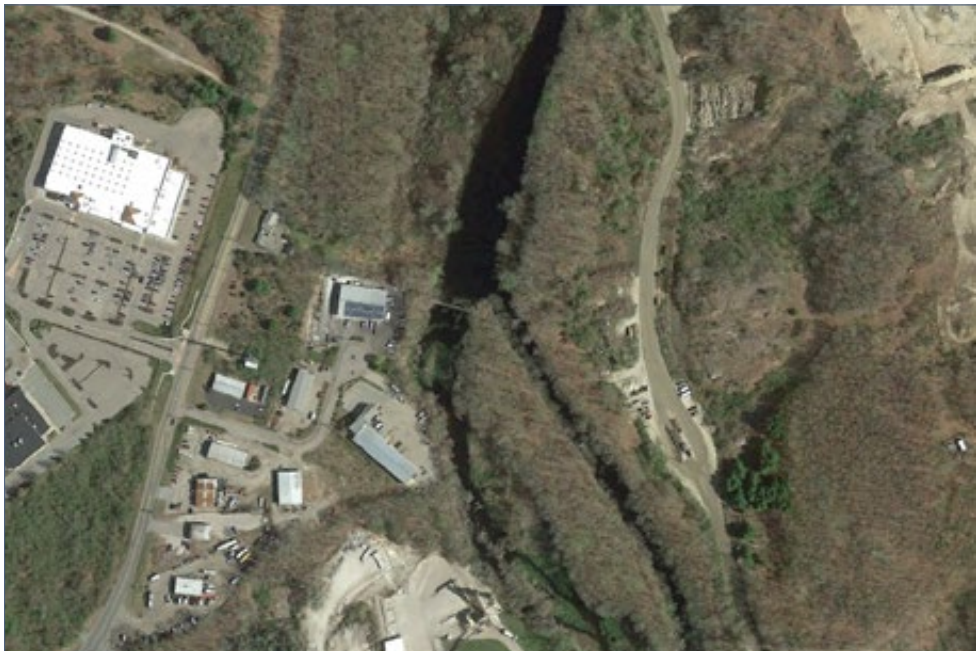
FIGURE 2.8-9 | White Rock Dam before removal, May 2015
