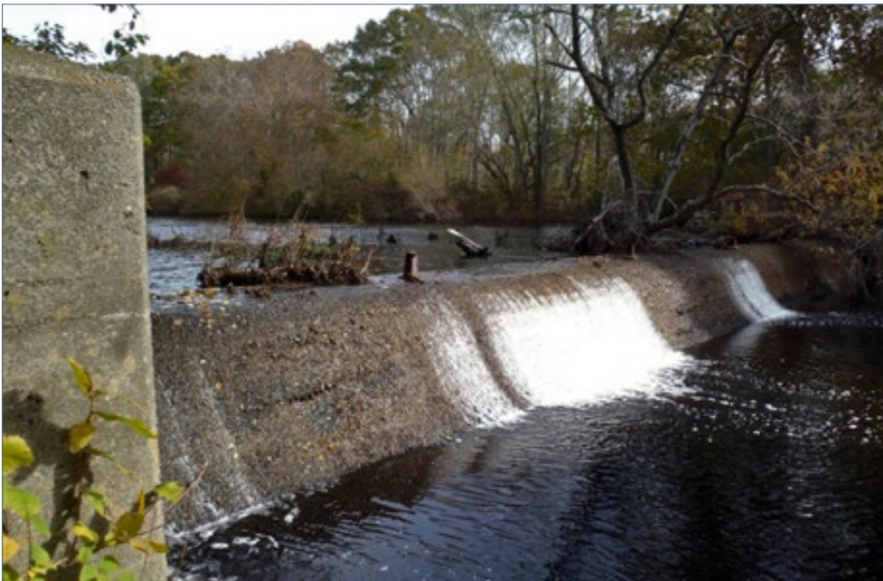
FIGURE 2.8-11 | White Rock Dam before removal
