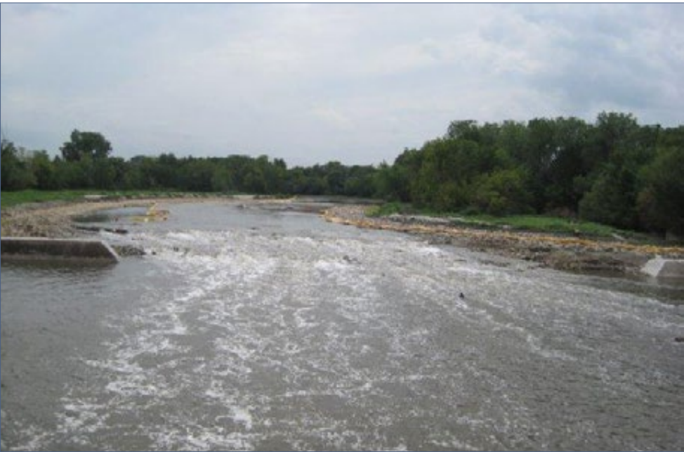
FIGURE 2.8-4 | Hofmann Dam after removal
