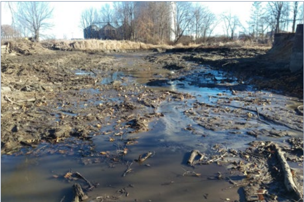
FIGURE 2.8-22 | A check dam was used to dewater the dam's backwater as the earthen portion of the dam was removed.
