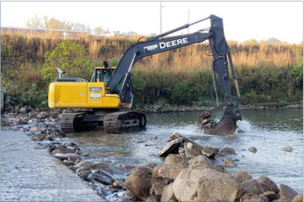
FIGURE 2.8-42 | An excavator is used to construct the riffle. October 10, 2019.
