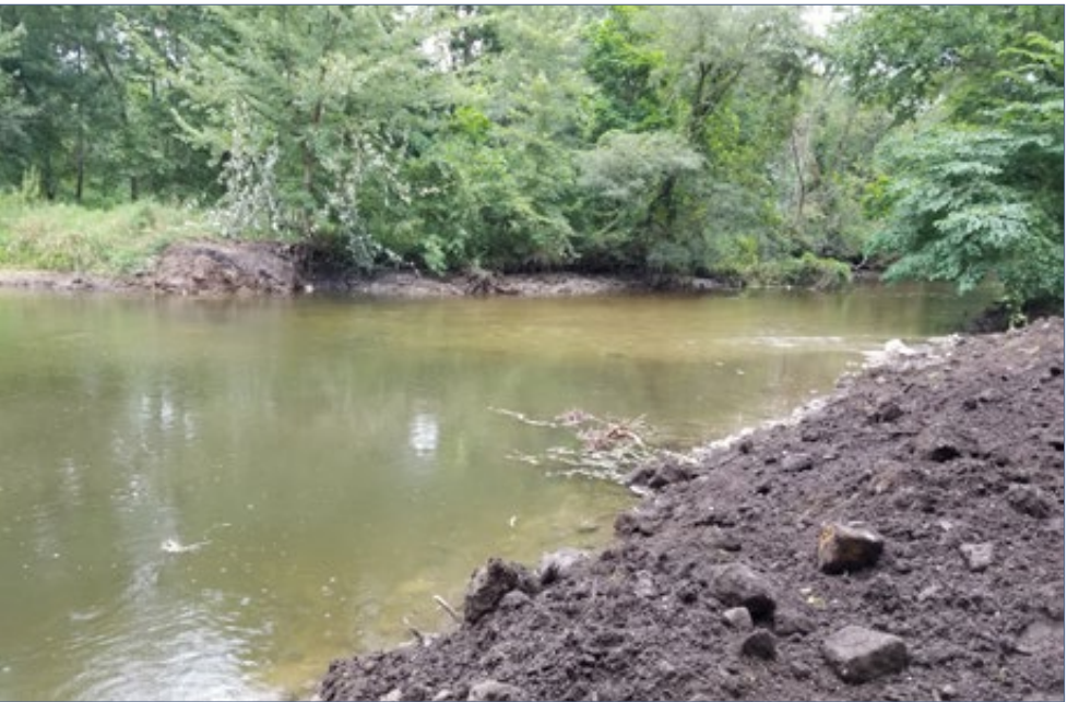
FIGURE 2.8-28 | Fox Farm Road dam after removal. August 15, 2018
