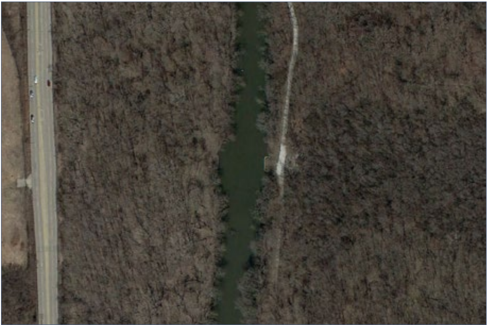
FIGURE 2.8-6 | Armitage Dam after removal.
