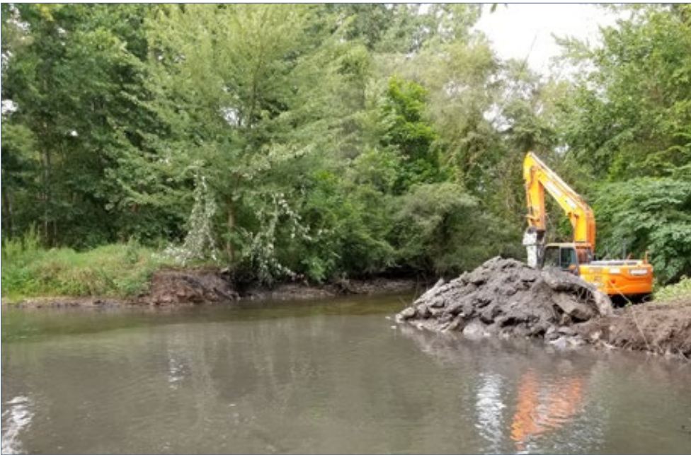
FIGURE 2.8-27 | Concrete and rebar is piled next to former dam location following removal. August 14, 2018.
