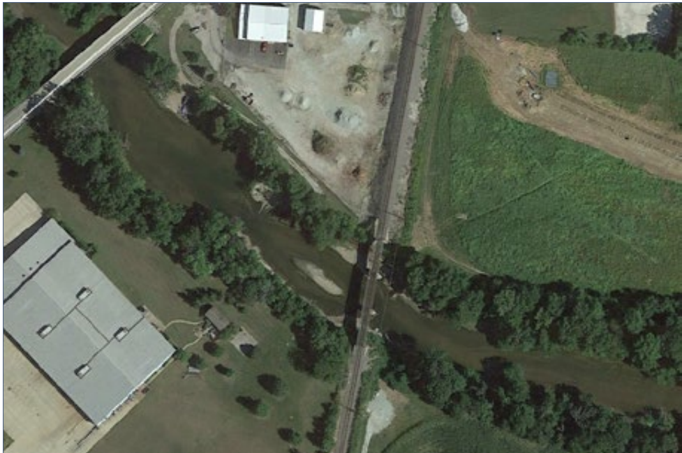
FIGURE 2.8-18 | North Manchester Dam after removal, August 23, 2013
