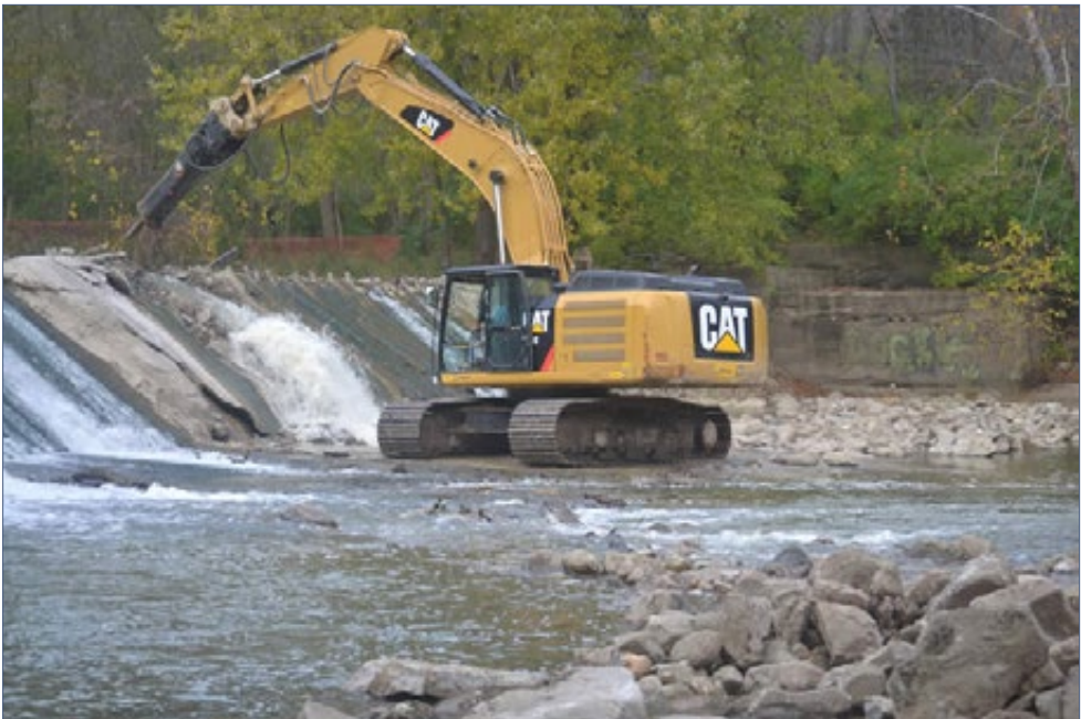
FIGURE 2.8-30 | The West Milton Dam is breached, or lowered 3 feet, to gradually release silt and save mussels upstream.
