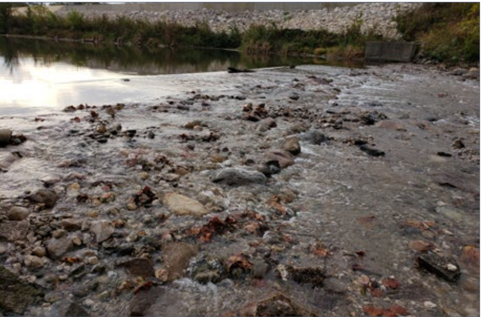
FIGURE 2.8-44 | Completed constructed riffle. October 11, 2019.
