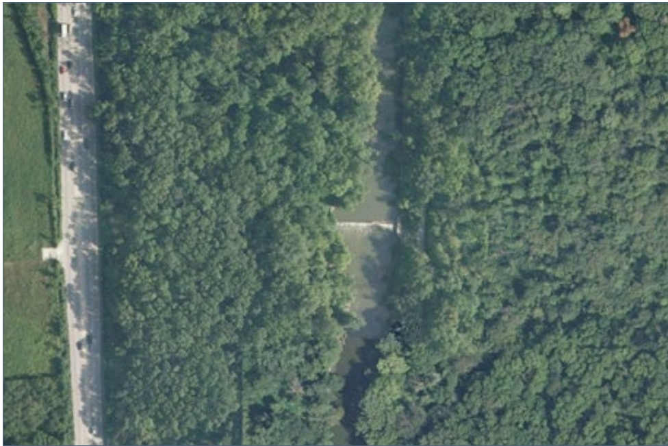
FIGURE 2.8-5 | Armitage Dam before removal.
