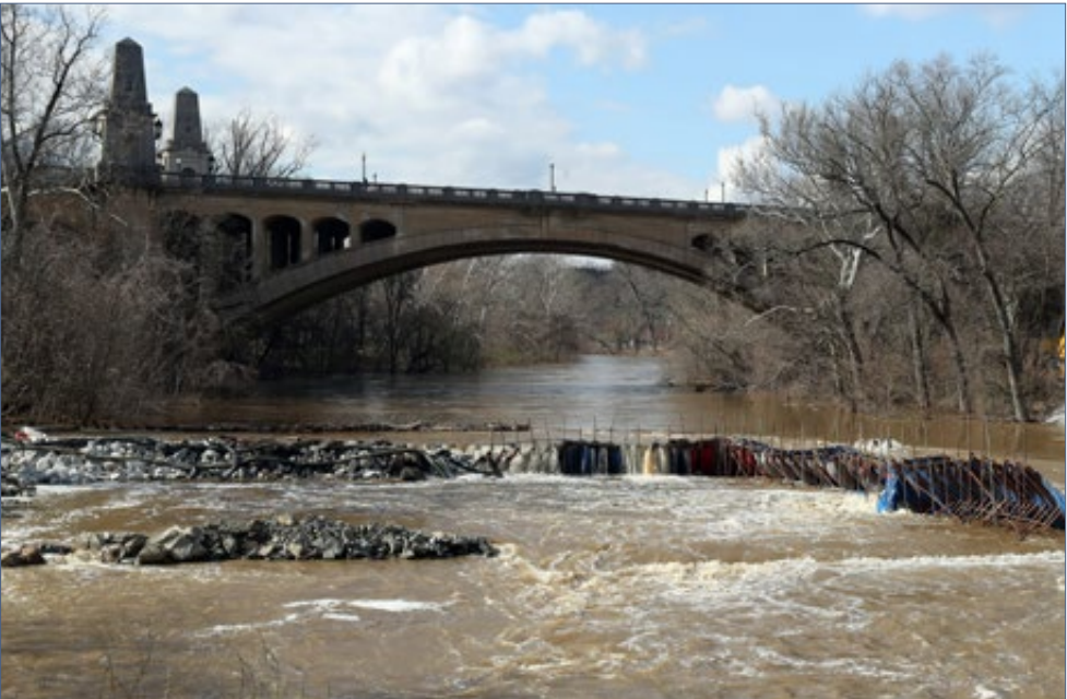
FIGURE 2.8-48 | Water is diverted around a low-head dam in Delaware during removal.
