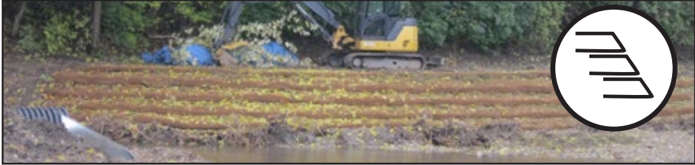
FIGURE 7.4-2 | Vegetated geolift
