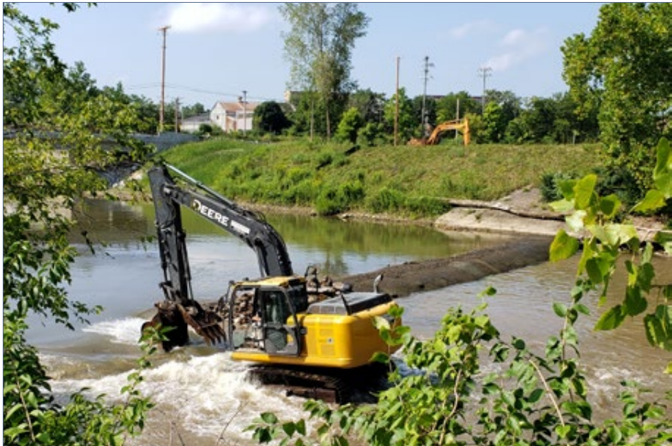
FIGURE 2.8-34 | Indiana Steel & Wire Dam during removal. August 19, 2019
