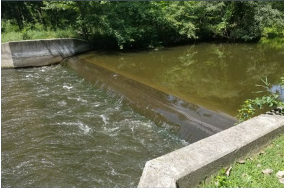
FIGURE 2.8-25 | Fox Farm Road Dam before removal, July 25, 2018
