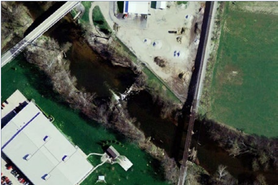
FIGURE 2.8-17 | North Manchester Dam before removal, March 30, 2005
