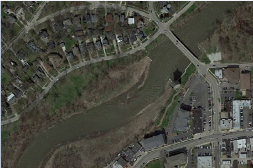
FIGURE 2.8-2 | Hofmann Dam after removal
