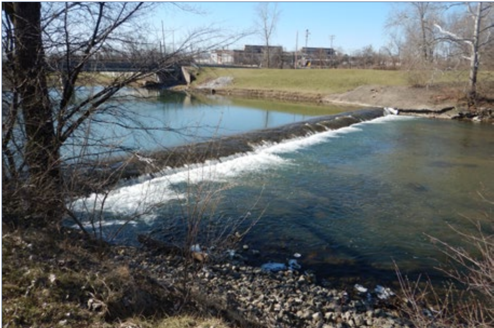
FIGURE 2.8-33 | Indiana Steel & Wire Dam before removal. March 16, 2017
