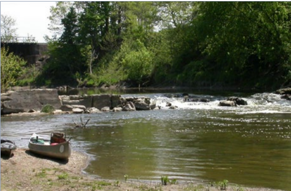
FIGURE 2.8-19 | North Manchester Dam before removal.
