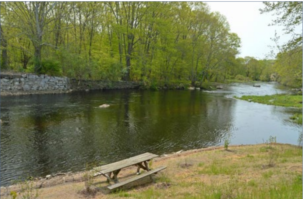
FIGURE 2.8-12 | White Rock Dam after removal
