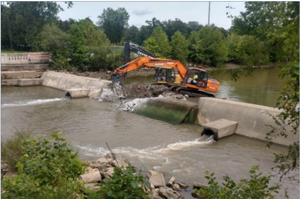
FIGURE 2.8-38 | The formerly clogged spillway pipes were cleared prior to removing the center of the dam.
