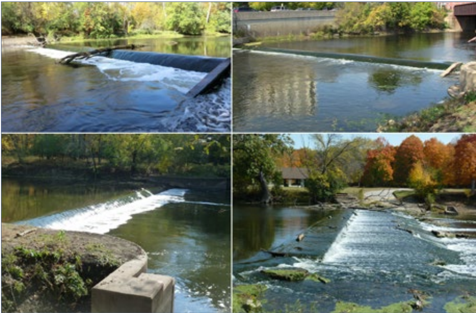
FIGURE 2.8-7 | Armitage Dam before removal.
