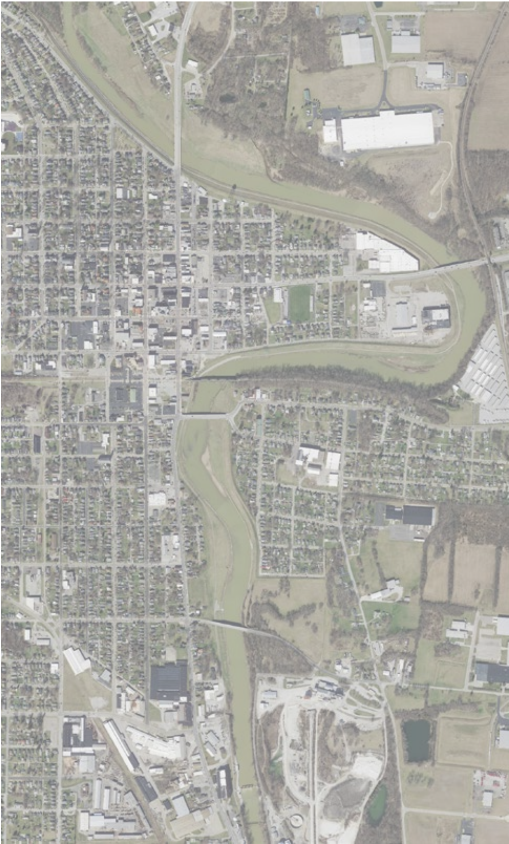
FIGURE 7.2-1 | Existing Conditions of the Piqua Dam Backwater
