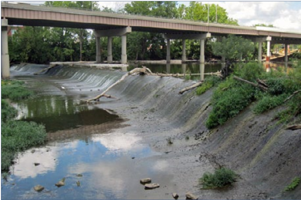
FIGURE 2.8-49 | 5th Avenue Dam before removal, October, 2011.
