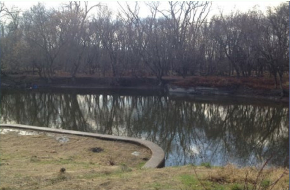
FIGURE 2.8-8 | Armitage Dam after removal.
