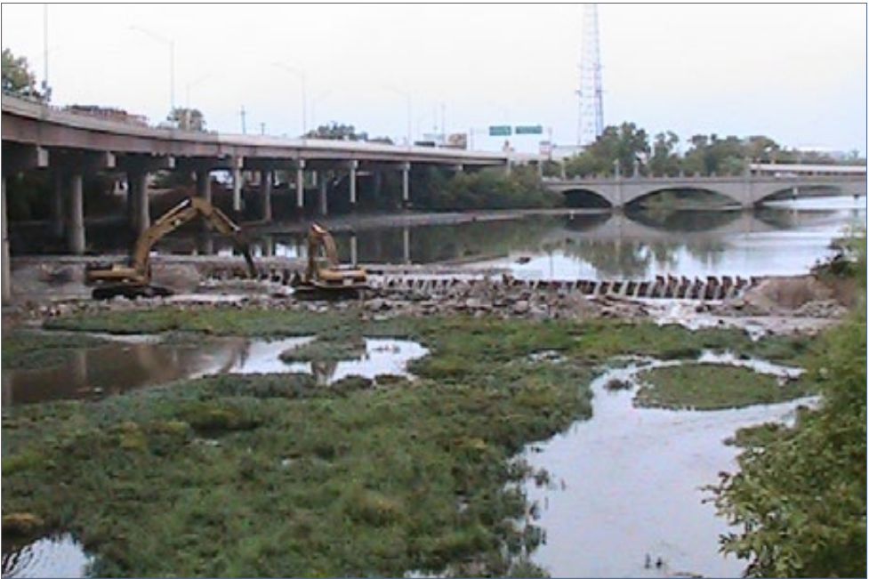
FIGURE 2.8-50 | Removal of the 5th Avenue Dam begins. August 30, 2012.
