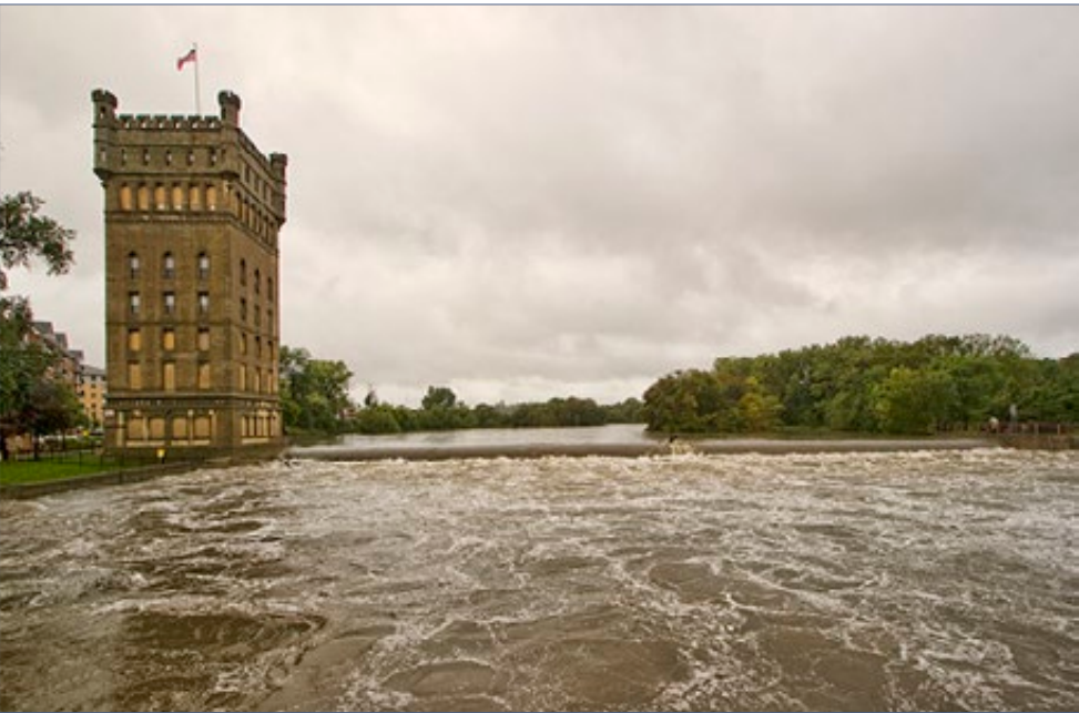
FIGURE 2.8-3 | Hofmann Dam before removal, April 7, 2017
