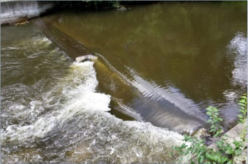
FIGURE 2.8-26 | Initial dam breach during removal process. August 10, 2018.
